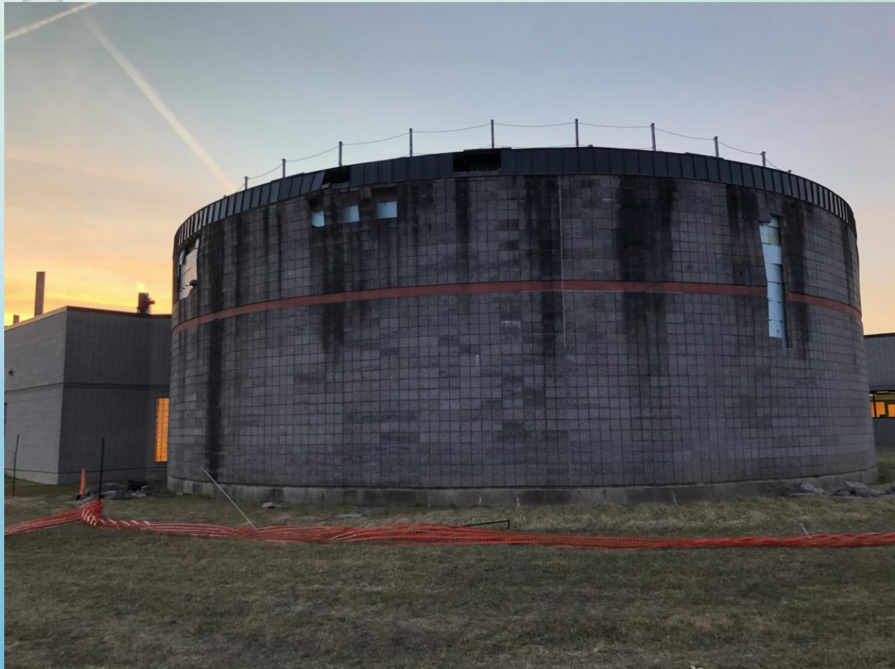
Milton St. – Primary Digester Wall
