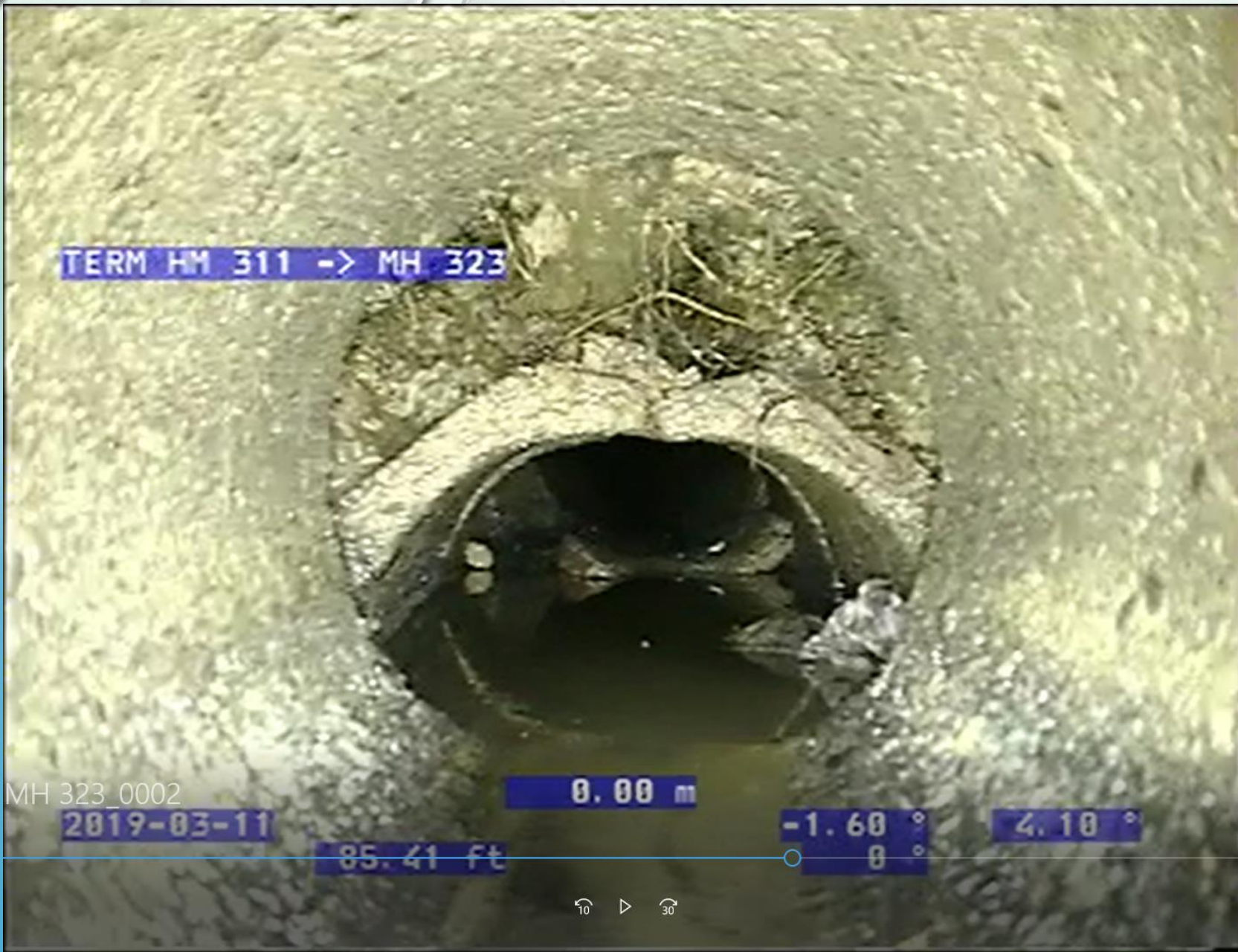
Irvine Pl. – City of Elmira – 2019 Road Program
